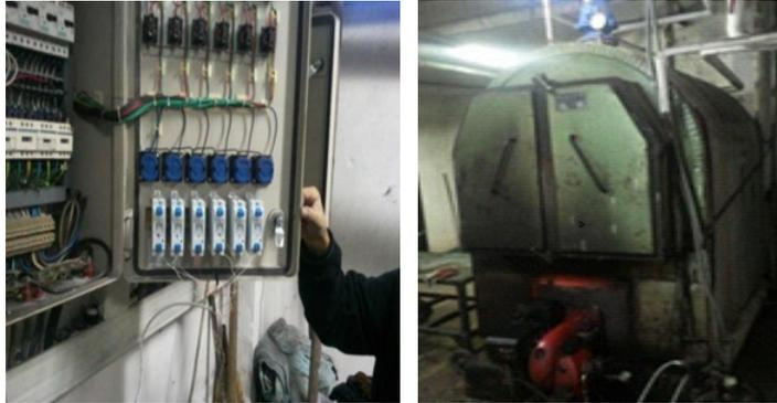
**Figure 7.** SSR driver table and the controlled heating pump
